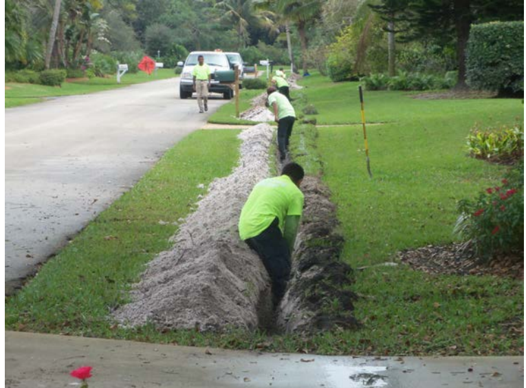
Contractor crews hand digging low pressure force main trench during construction.
