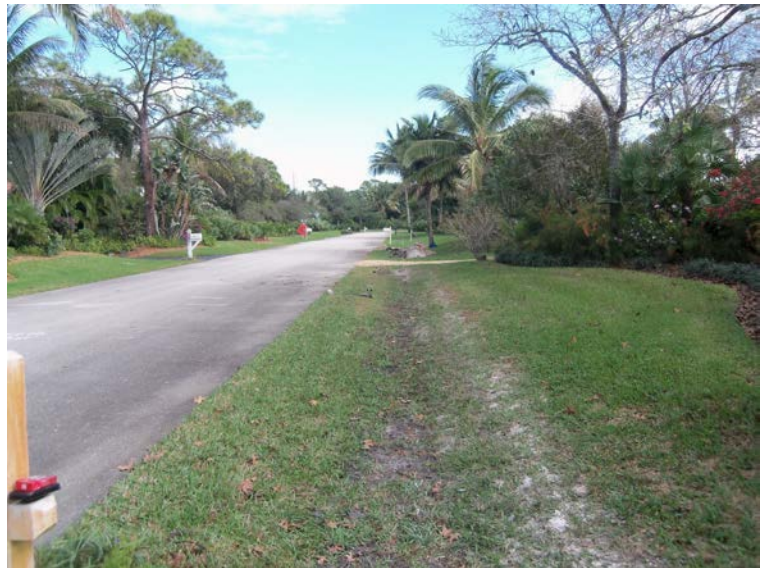
Restored trench after installation of the low pressure force main.
