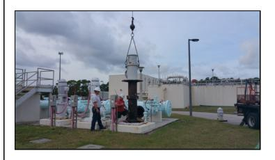
**LEFT.** Filter pump station #2, pump #3 has been removed for inspection and overhaul. Removing the pump allows for a thorough inspection to determine pump condition for need of repairs to worn and deteriorated parts. This helps to prevent unexpected failures.
