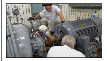
**RIGHT.** The maintenance team has added shims to a blower motor as indicated with the new laser alignment tool.
