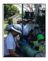
**LEFT.** The District Construction crew performed the scheduled replacement of the 8 inch plug valve at IQ site 505 (Turtle Creek) metering station.
