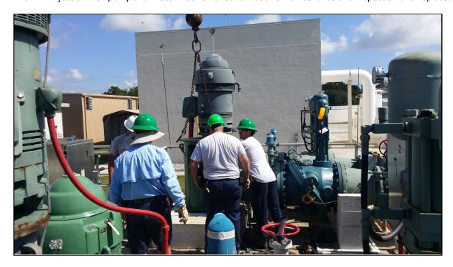
**BELOW.** One of four check valves was removed and sent to our on-site pump repair shop. We have a standby unit so that we can take out one of the four check valves and install the standby unit to have the capability of full capacity while we are servicing the removed unit.
