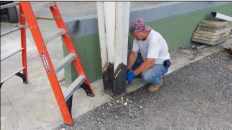
**BELOW.** The District is preforming routine maintenance on one of our clarifiers. The Maintenance Crew has stripped the exterior of the stilling ring to bare metal and is applying a galvanized treatment to ensure several years of service.
