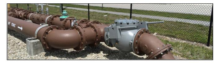
**ABOVE**. The District Construction Crew performed the scheduled replacement on the Nano Concentrate Filtration force main check valve from the Town of Jupiter Water Treatment Plant.
