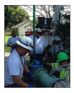
**LEFT.** The District Construction crew performed the scheduled replacement of the 8 inch plug valve at IQ site 505 (Turtle Creek) metering station.
