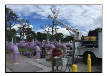
**LEFT.** At plant site, IQ 511; Master Reclaimed Water pump station with the District Construction crew performed the scheduled task of replacing a 14 inch check valve with a spare.
