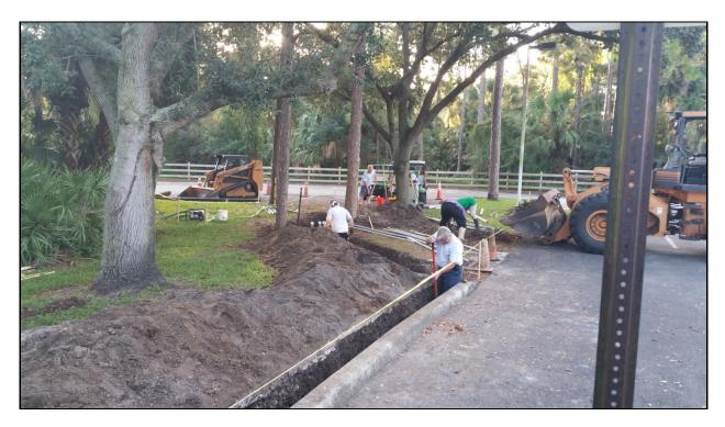
The pad has been poured and the electrical conduit is buried and landscaping restoration is under way.
