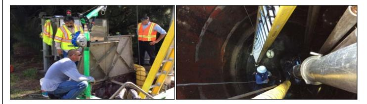
**RIGHT.** In the Jupiter Hills development, two (2) lift stations, #52 and #59, worked on the process of installing new control panels, electrical disconnects/grounding, and a stantion rack.
