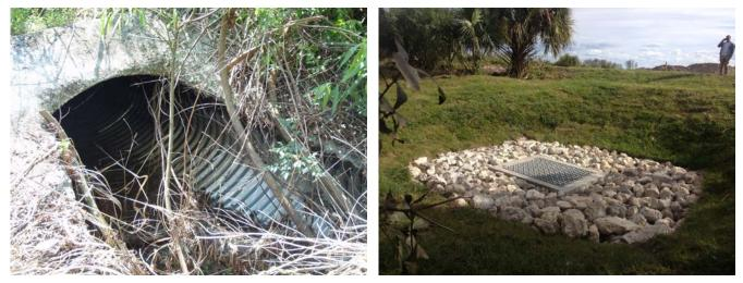
The culvert pipe that was the sampling station 88 (left) at Sonoma Isles (previously Parcel 19), and the newly completed water control structure (right). This station drained the former agriculture site with high Phosphorus loads. The new drainage feature is connected to a wetland treatment area and will only discharge during extreme rain events. This should improve water quality at this site.
