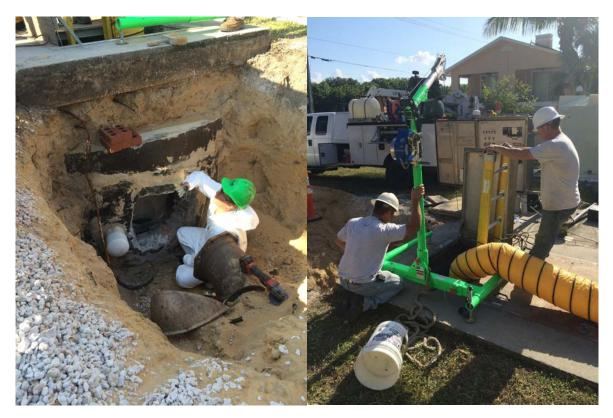
*Lift Stations 57, 58, 62, 65, 66, 68, 94 and 97:* Staff are systematically working in these areas to locate or install right of way clean outs in coordination with upcoming TV inspections.
